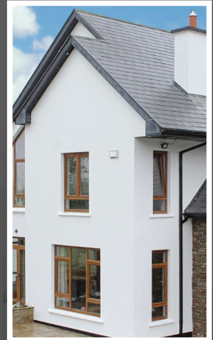
EXTERIOR PAINTING WITH DIRT-RESISTANT PAINT
