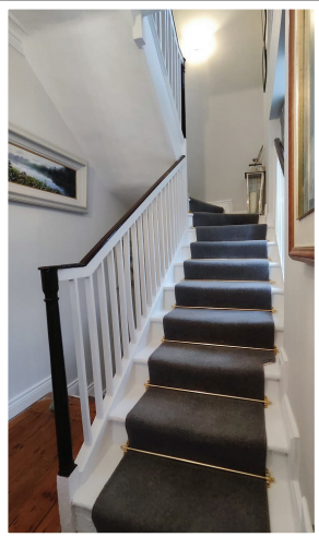
HALL & STAIRCASE RENOVATION
