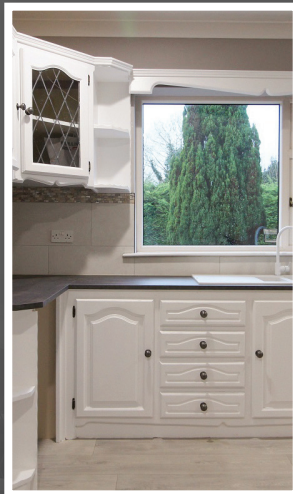
KITCHEN REMODEL WITH NEW WORKTOP
